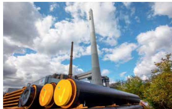
Preparations for the link are underway ...
