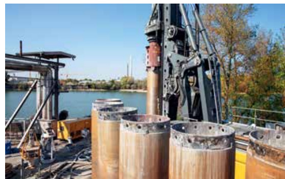
... and are progressing at full steam
