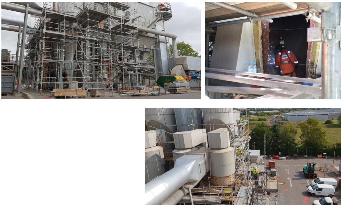
Figure 10 - Access to and upgrade of the flue gas treatment plant
