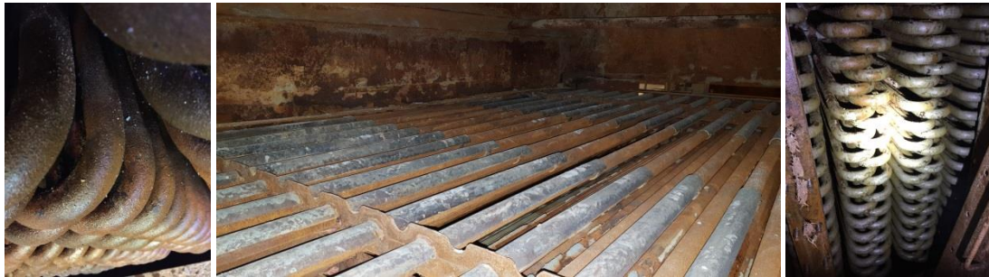
Figure 6 - Heat exchanger bundles after cleaning
