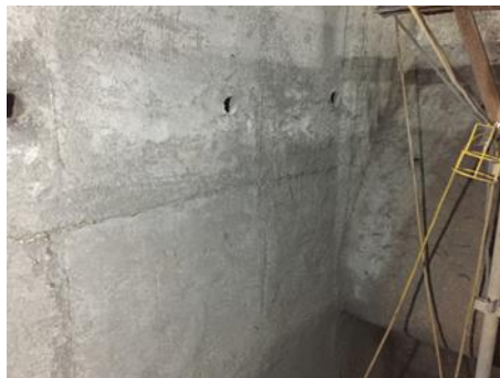
Figure 2 - New refractory (insulating layer) following application.
