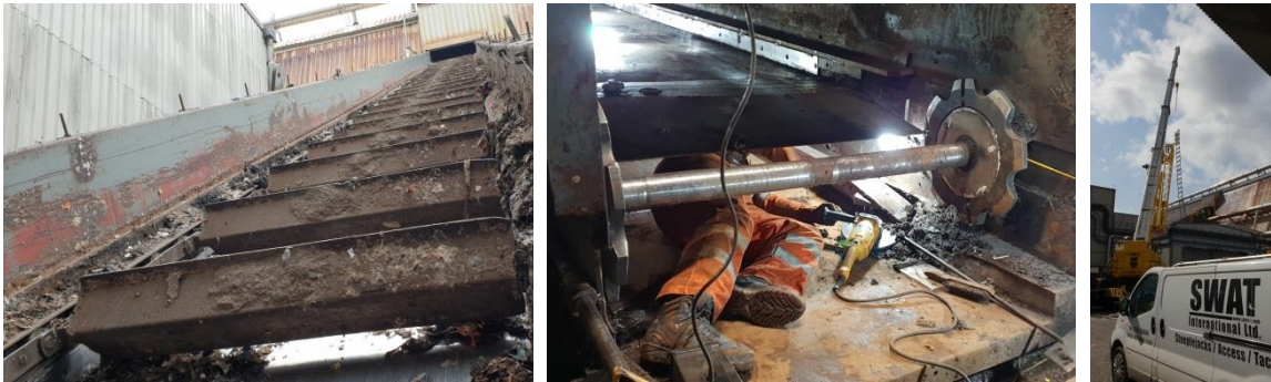
Figure 3 - Worn chain, work inside the conveyor and new chain being installed.
