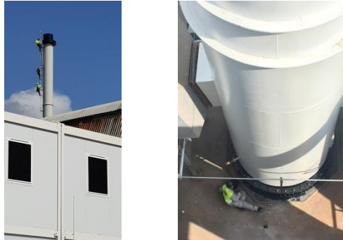
Figure 11 - Steeplejacks inspecting and painting a stack
