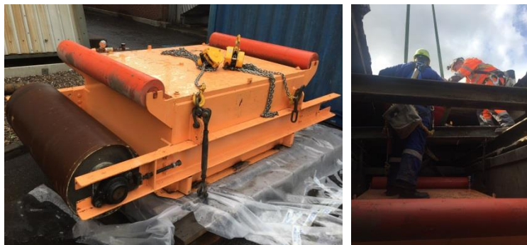
Figure 5 - Magnet reinstallation
