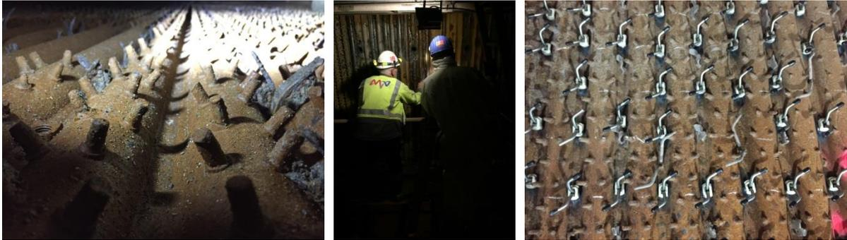
Figure 1 - Boiler tubes after hydro demolition, MVV staff inspecting tubes and new refractory anchors in place ready to be coated.
