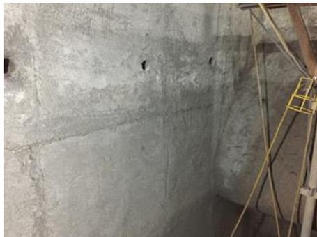
Figure 2 - New refractory (insulating layer) following application.
