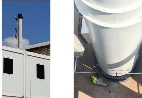
Figure 11 - Steeplejacks inspecting and painting a stack
