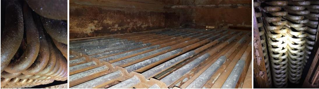
Figure 6 - Heat exchanger bundles after cleaning
