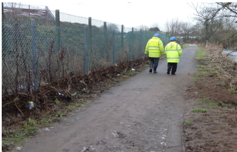
Figure 12b: Wrack marks would suggest a potential depth of 0.3-0.4m across the left bank footpath at location 6, Figure 6 (Arup, 19/1/16).
