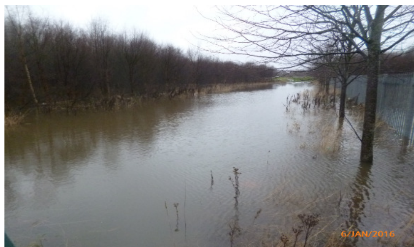
Figure 8a: Flooding along BMX track access road off Forties Road on 6/1/15 (photo courtesy of DCC), approximate depth 0.2m. Location 2, Figure 6.
