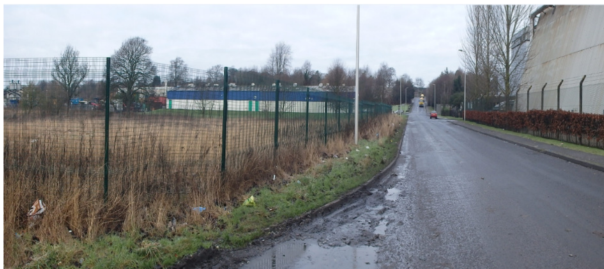
Figure 9c: Silt deposited in layby opposite recycling centre (19/1/16 – 12 days after flood, Arup)
