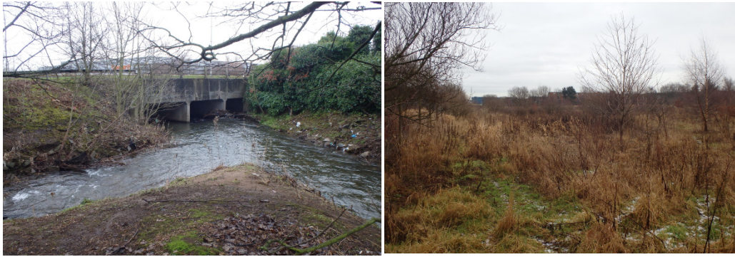
Upstream face of the bridge under Baldovie Road
