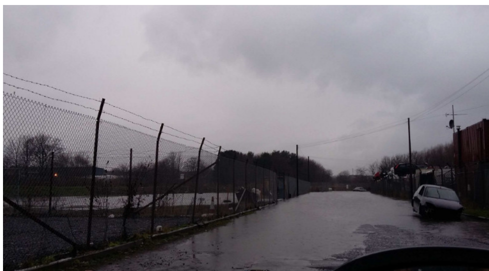
Figure 11a: Flooding on Beryl Street to south of scrapyard showing scrapyard on left of photo (date unknown, image courtesy of Michelin). Location 6, Figure 6.
