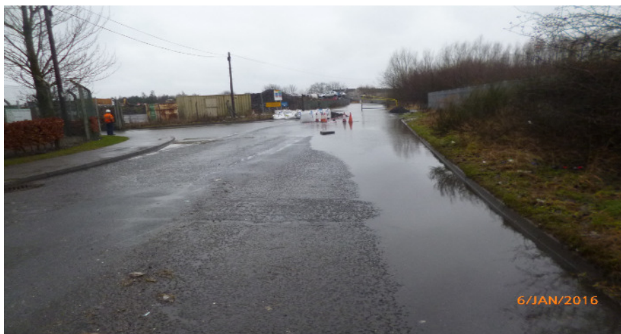
Figure 9a: Forties Road flooding on 6/1/16, showing the entrance to the recycling centre on the left and the scrapyards to the left of the road in the distance. Forties road was inundated to approximately the recycling centre entrance (image courtesy of DCC). See location 3 on Figure 6.
