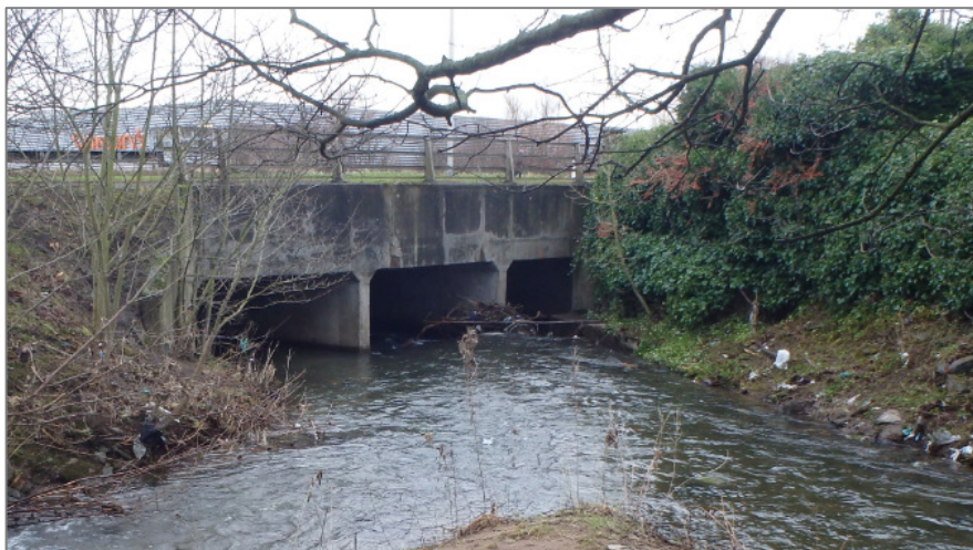
Figure 8. Upstream face of the B978 Bridge. Note the confluence of the Dighty Water and Fithie Burn immediately upstream.
