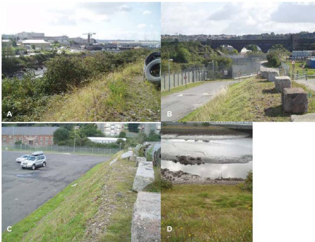
(a) east-side (b) north-side (c) west-side (d) south-side
