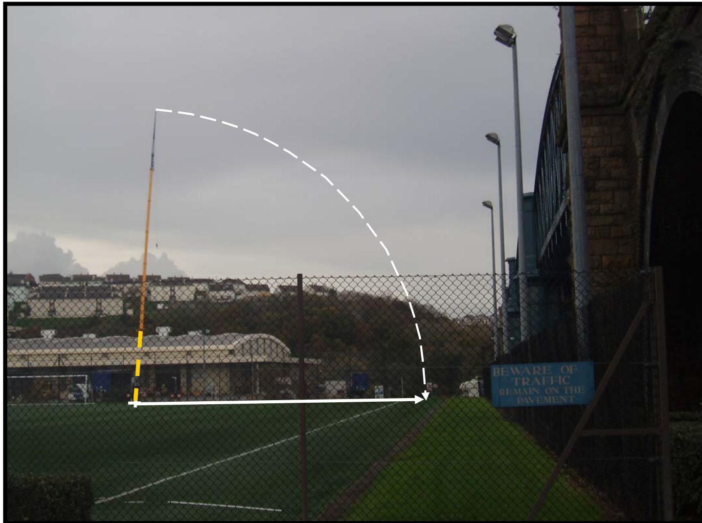
Figure 2 Chimney Stack and Network Rail Track
