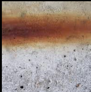
iron filing rust on concrete
