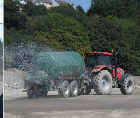
Damping down on site to minimise dust
