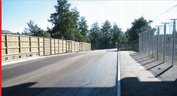
The acoustic fence along the new access road that will reduce noise disturbance as vehicles enter and leave the facility.
