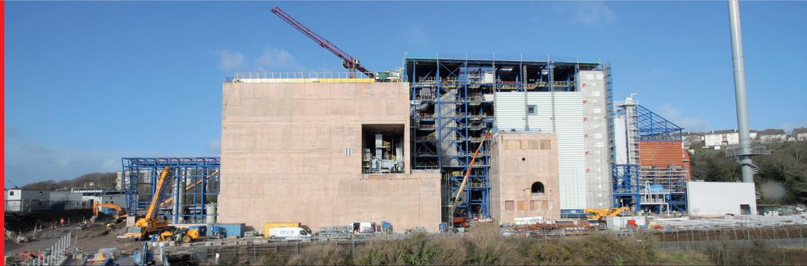
New features that can be seen in this recent photograph from our webcam include the blue steelwork for the water treatment plant on the left-hand side, the arched aperture for the steam pipe in the wall of the turbine hall and the chimney.
