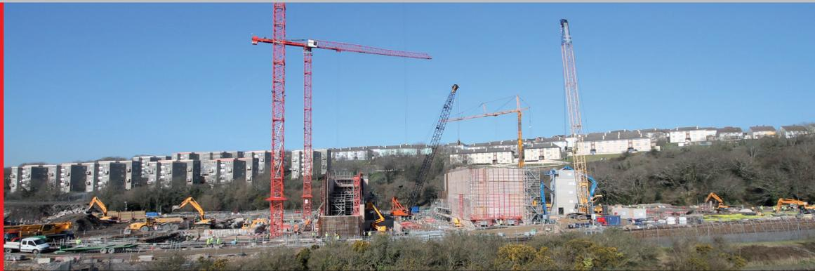
This picture, taken from our webcam, shows the progress on site. Currently, the first walls for the turbine hall and the waste bunker are being erected.
