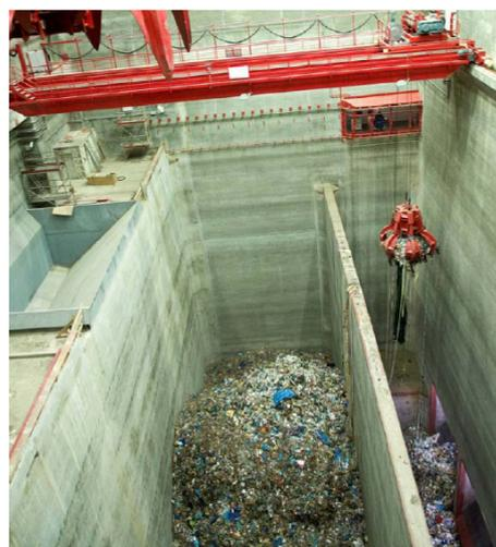
**Photograph 2: Typical bunker view with crane control cabin (background), tipping chutes (right), stored waste (centre) and feed hopper (left, flap gate closed)**
