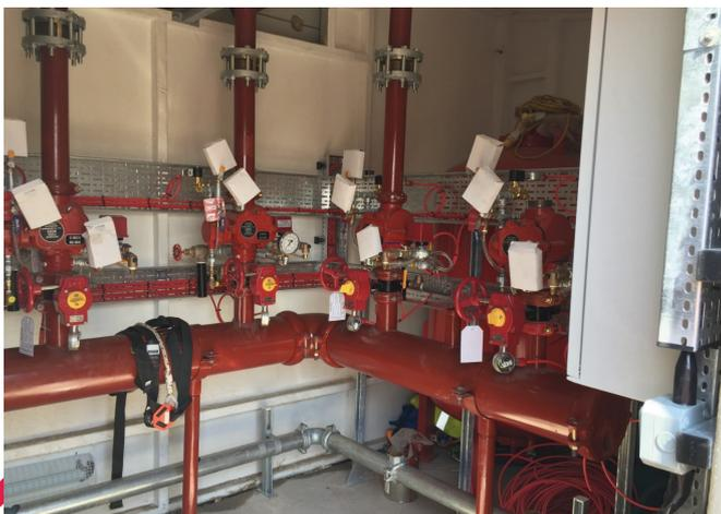
Fire protection manifolds installed
