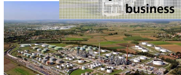
Joint district heating project in Ingolstadt
