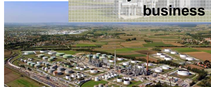
Joint district heating project in Ingolstadt
