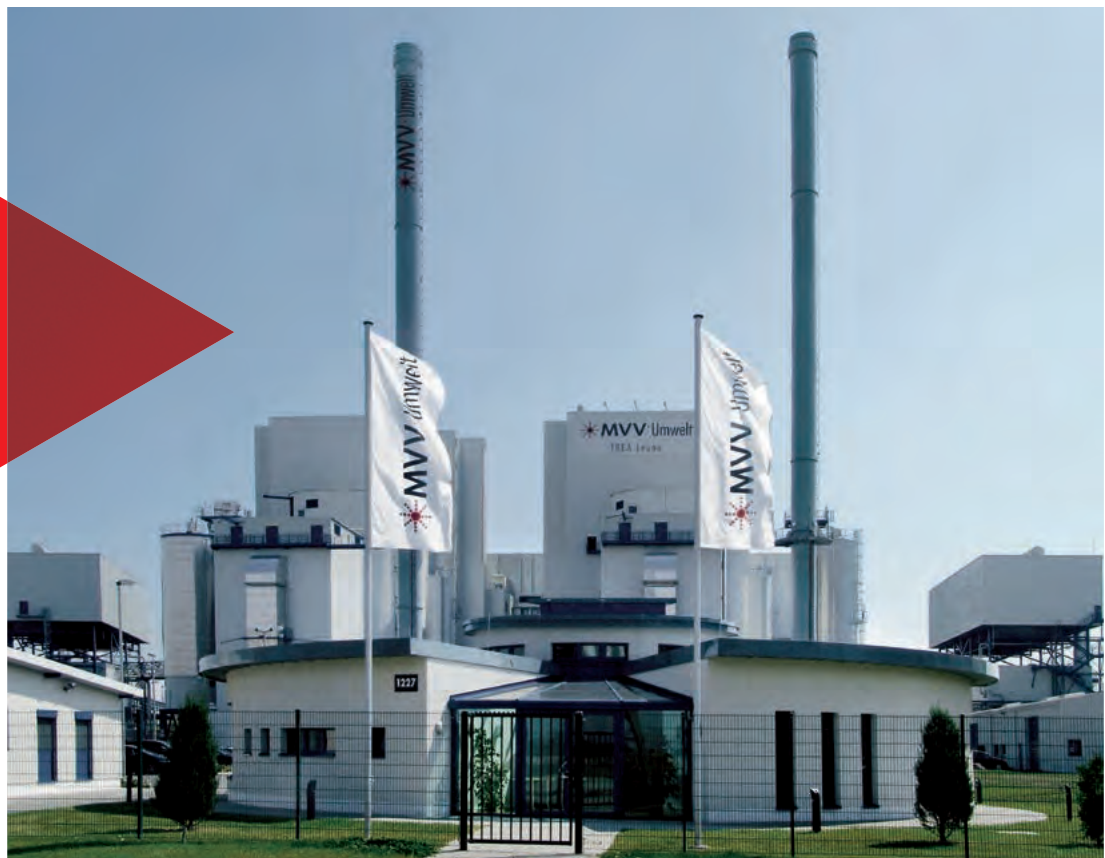
OUR ENERGY FROM WASTE PLANT IN LEUNA
