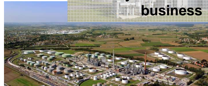
Joint district heating project in Ingolstadt
