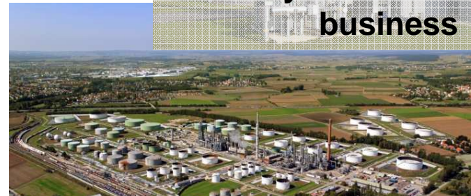
Joint district heating project in Ingolstadt
