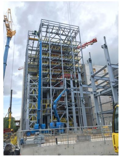
FGT: Flue gas duct sections and conveyors in place
