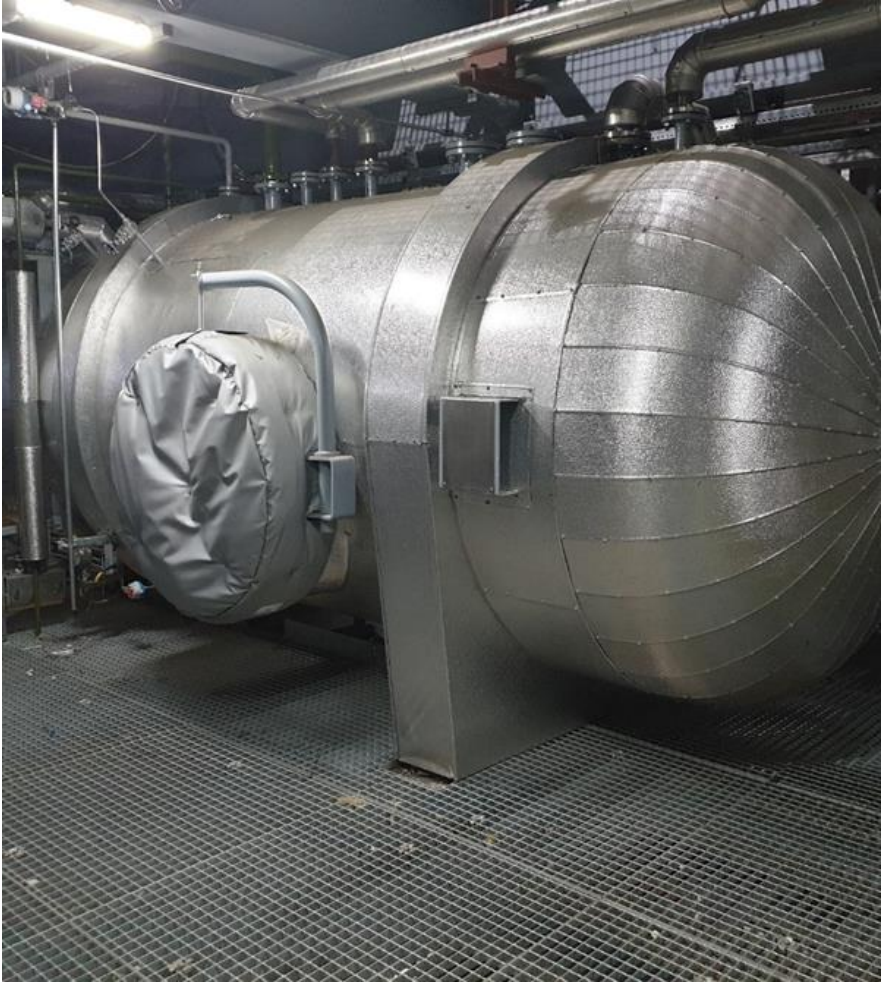
SPG Insulation and Cladding Works completed
