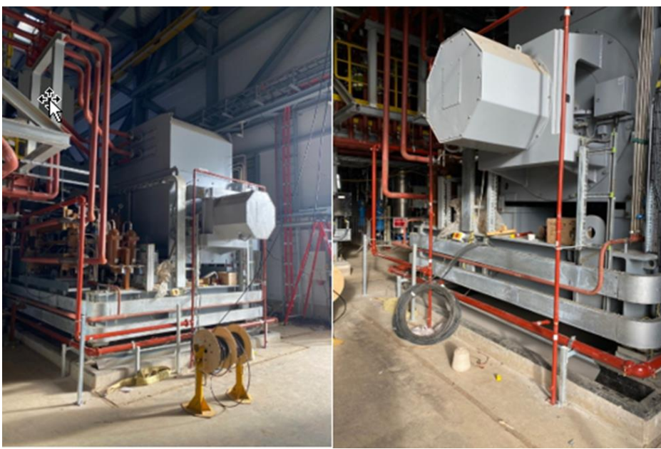
Turbine Hall – Sprinkler Installation around Turbine Generator Unit
